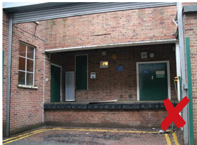
With a ceiling and three walls, smoking would not be permitted on this loading bay
